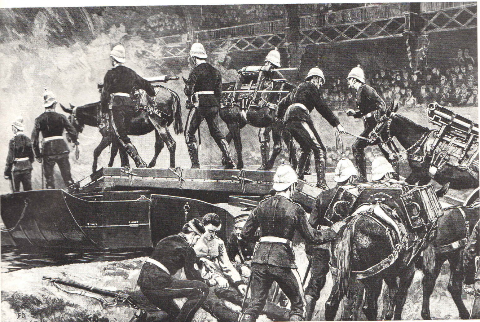
A mountain battery demonstrates to the public its skill at crossing a stream by pontoon bridge.
